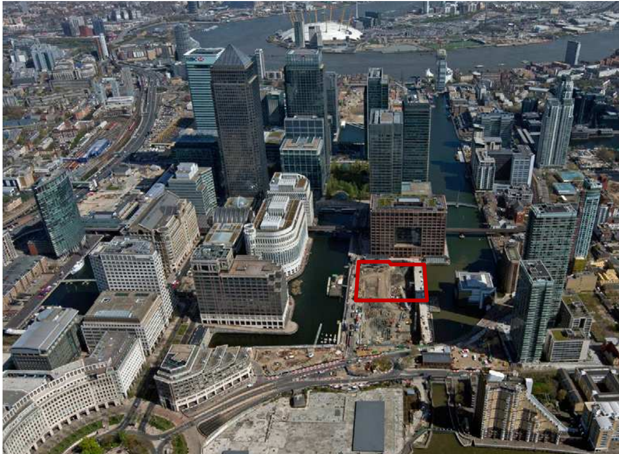
Figure 3 – Aerial view of the site, looking east.
